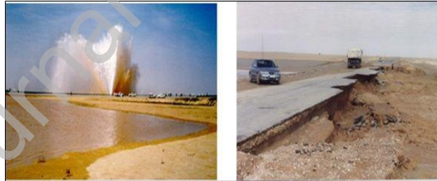
Figure 1: Pipe rupture and damage at the MMRP.
