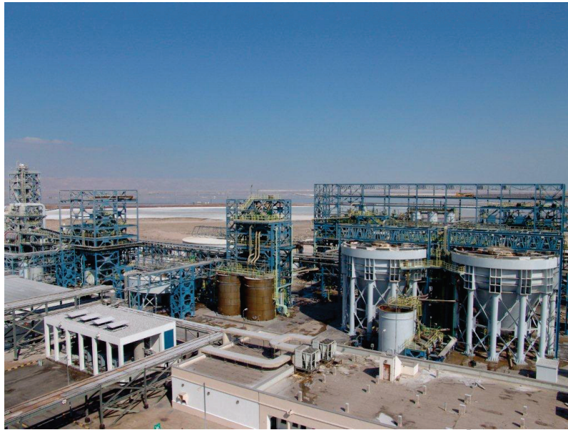
Figure 2: APC extraction and refinery facilities – Dead Sea
