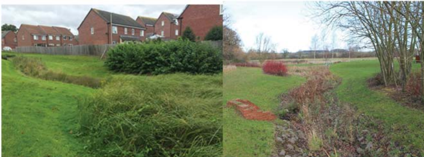
Figure 9.3 Example of a SuDS system, comprising of rock-lined swales and vegetated detention ponds, in Leicester, England. ©CraigLashford.
