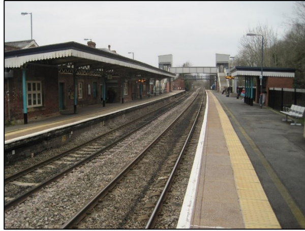
Figure 3.1: Leominster station site, Herefordshire, UK (Wikipedia, 14 March 2015.)
