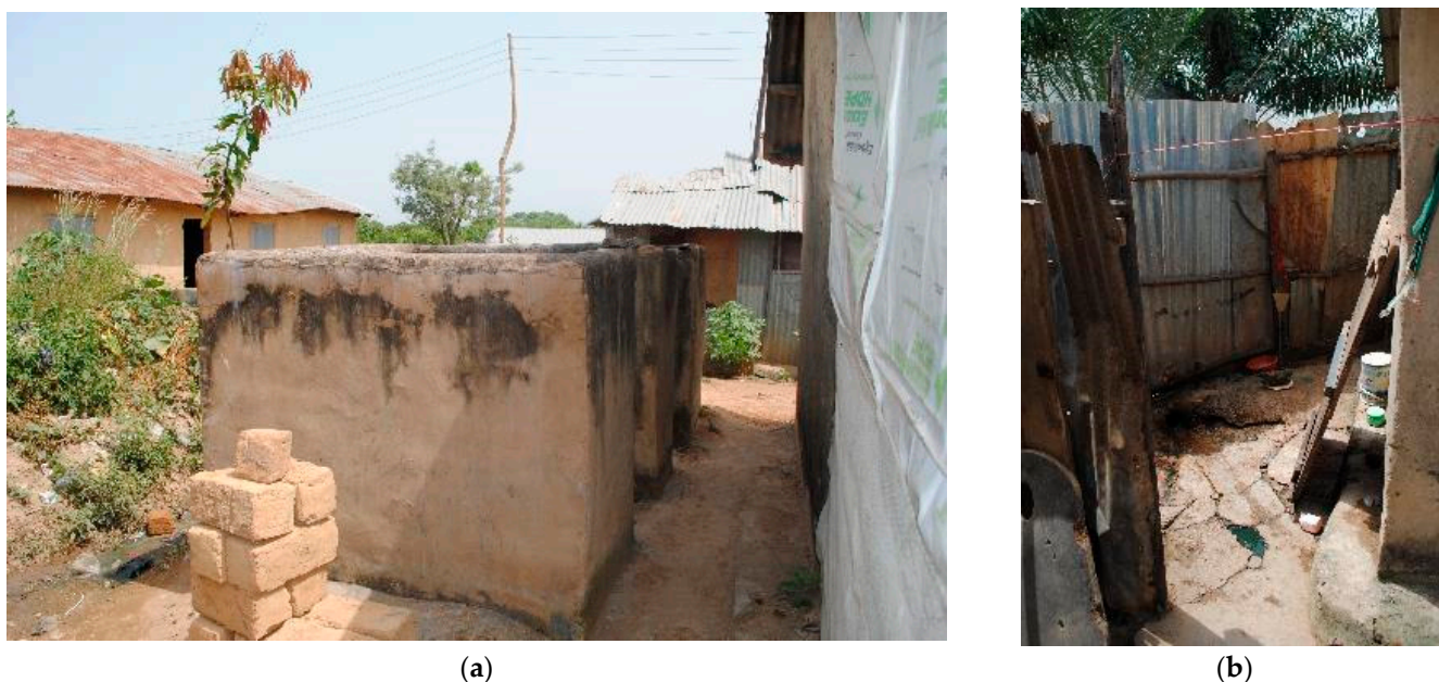
Figure 6. (a) Outdoor toilet and bathroom. (b) Outdoor bath area.
