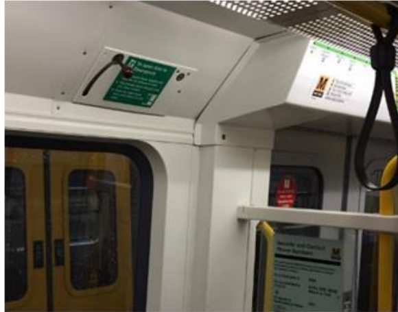
Figure 5: Manual emergency door handle on-board metro car 4067
