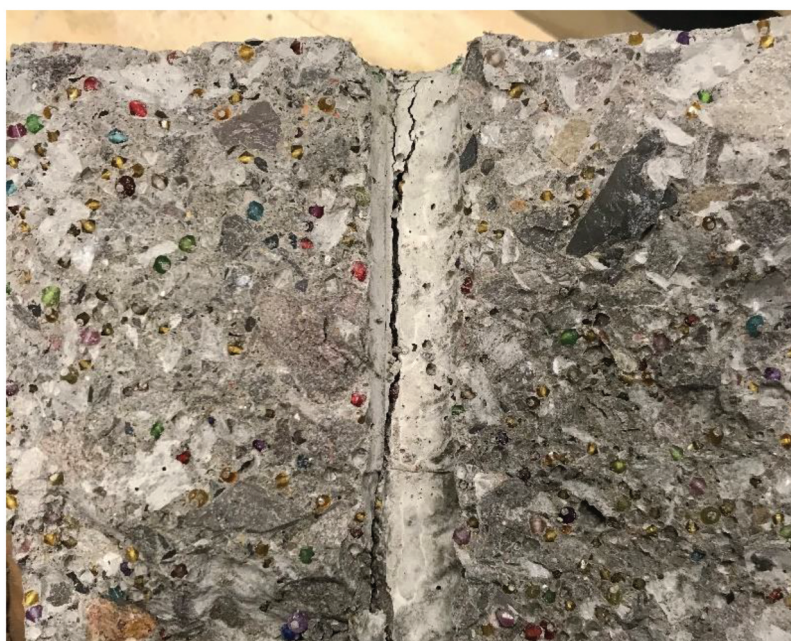
Figure 12. Steel-Concrete Interface After Failure (10% Replacement), illustrating the interface between the steel reinforcement and the concrete specimen for a 10% push-out sample after failure.
