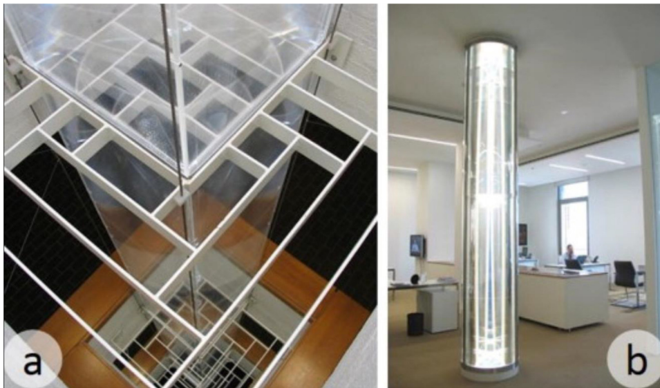
Fig. 8. (a) Light ducts penetrates building vertical voids and (b) side emitting ducts reproduced with permission [153].
