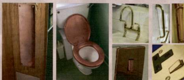
Figure 1. Examples of copper items (door push plate, toilet seat, tap handles, grab rails, door pull handle, light switch, socket)
