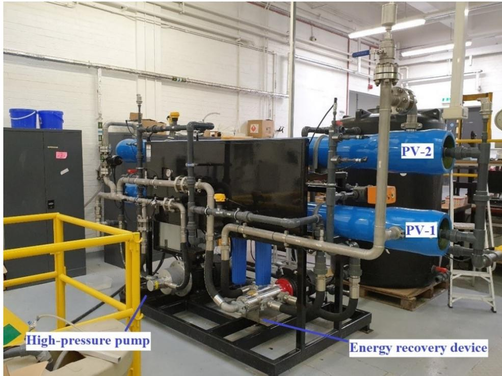
**Fig. 3.2.** RO system installed in the laboratory (front).
