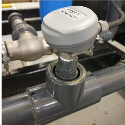
**Fig. 3.15.** Temperature transmitter.
