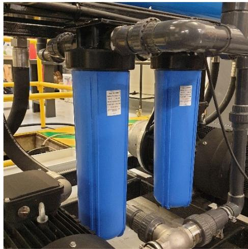
**Fig. 3.6.** Cartridge filters.
