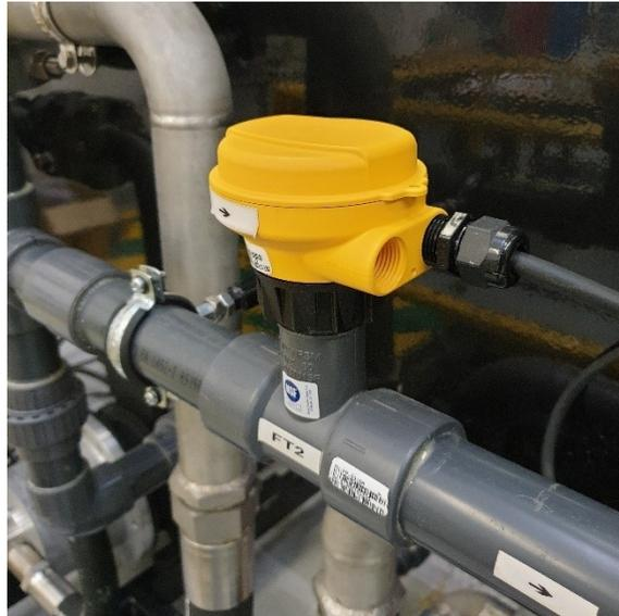
**Fig. 3.12.** Paddlewheel flowmeter.
