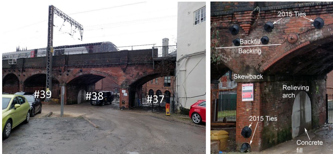
Fig. 1 Left—Northern view of the Marsh Lane Viaduct in Leeds, UK. Right—Closer view of the pier between Arches 38 and 39, showing the 2015 retrofit
