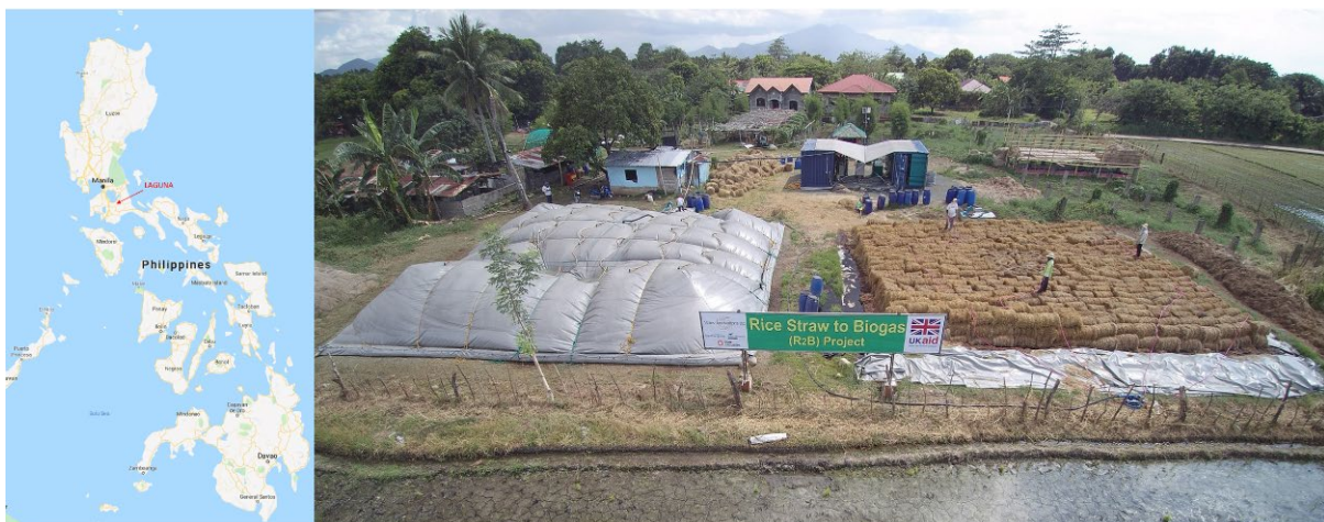
Figure 1 Location of Laguna (map adapted from Google Maps) and image of R2B pilot facility in San Francisco, Laguna, Philippines. The picture shows the two 500\text{m}^3 digesters (Left: digester covered with grey canvas and digesting rice straw. Right: preparation of digester with rice straw bales).
