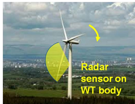
Fig. 1: The concept of compact radar sensors for WT structural monitoring.
