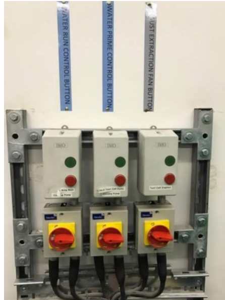
Figure 3.15: Main switches for cooling water pump and exhaust gas fan (Aston University mechanical engineering laboratory).
