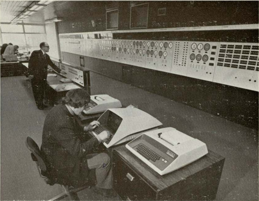
PLATE I WEST MIDLAND GAS CENTRAL CONTROL ROOM
