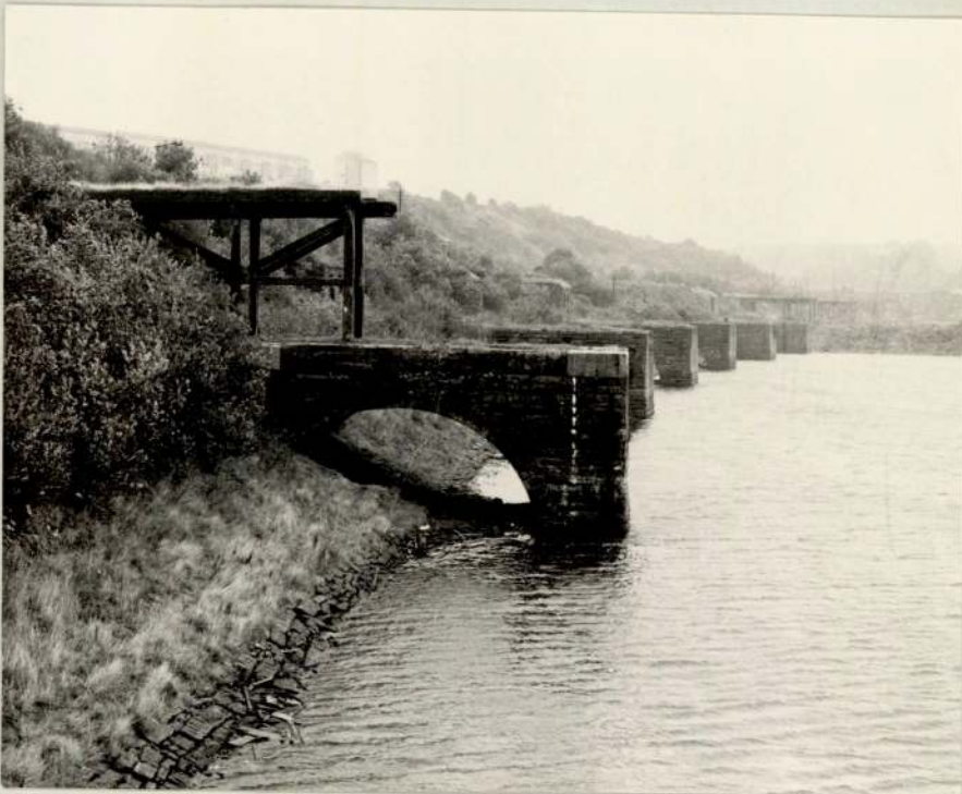
Fig. 7.17 Derelict staithe at Penarth Dock
