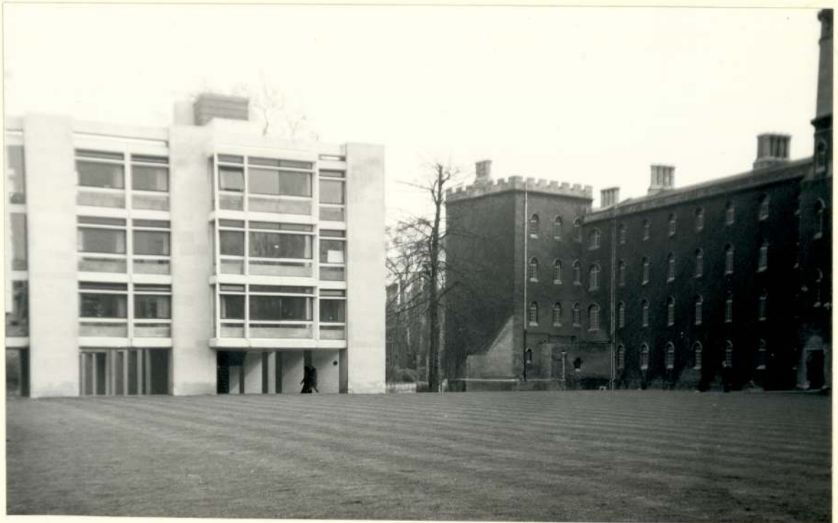
Plate No. 5.2 Cripp's Building, St. John's
