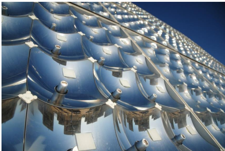
Fig. 5: Concentrated solar plant built near Tecate Mexico [Permission to reproduce from 32]
