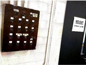
Figure 1: Engine area lights switches
