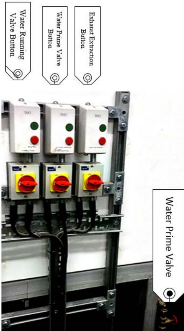
Figure 46: Water and exhaust extractions control keys.
