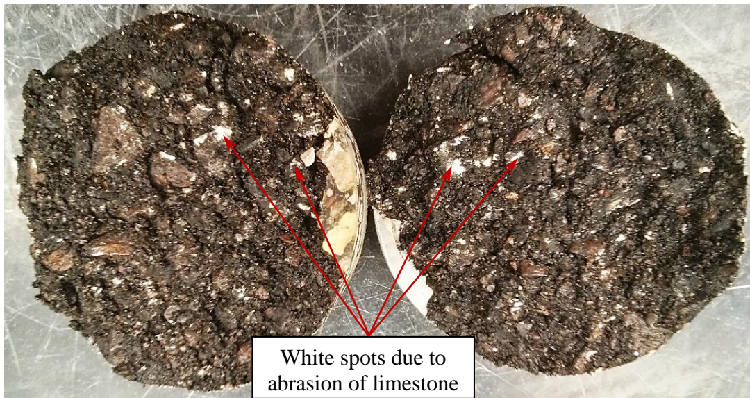
Fig.10 White spots due to abrasion of limestone aggregates on shear failure surfaces of asphalt concrete
