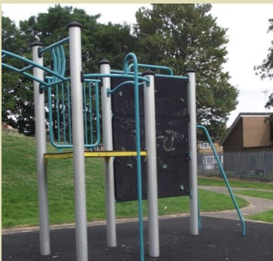
Figure 8: Graffiti at Kingshurst Park
