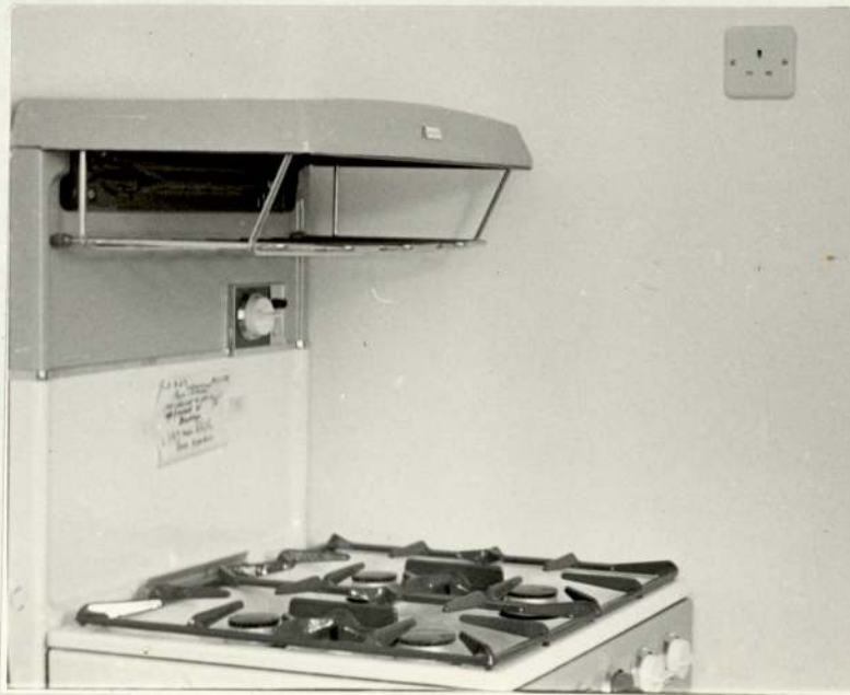
Plate 16.1 Badly positioned socket outlets. Cookers also badly positioned (top left) by doorway, (bottom) in corner of room.
