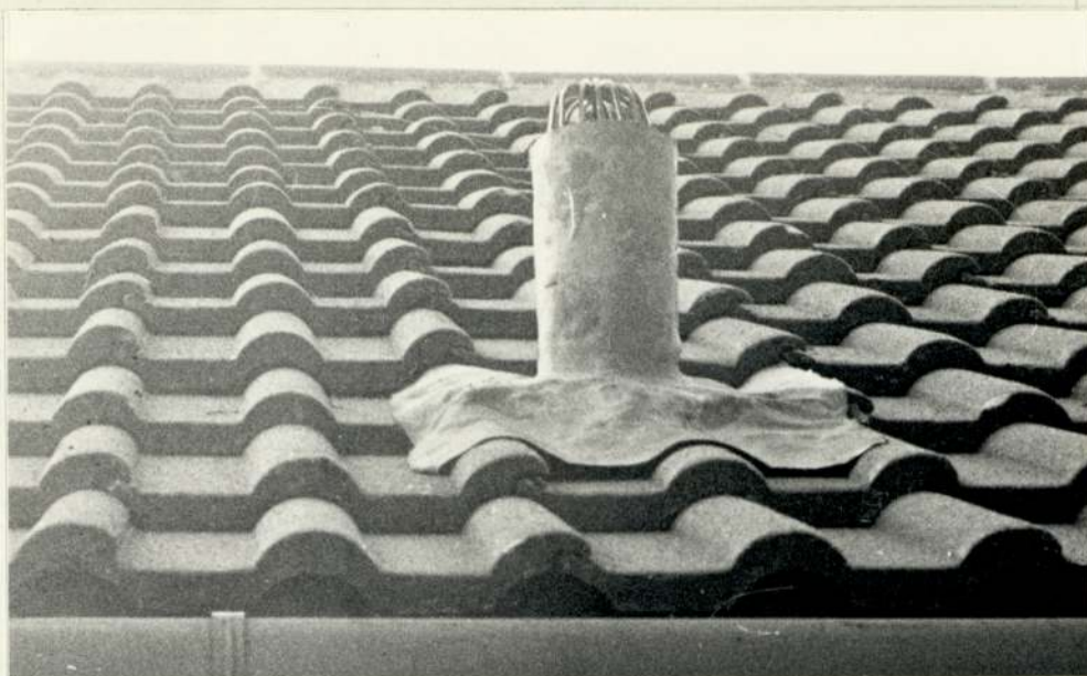
Plate 18.4 Lead slate not dressed down over tiles
