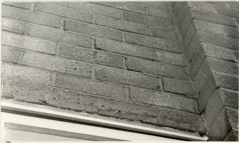
Plate 2.1 Cracking above ground floor window (Note the poor finish of the lintel)
