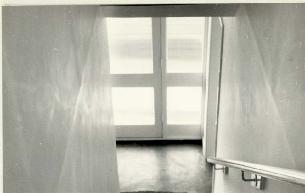
Plate 18.8 Unsightly joints between partitions of brickwork and plasterboard.
