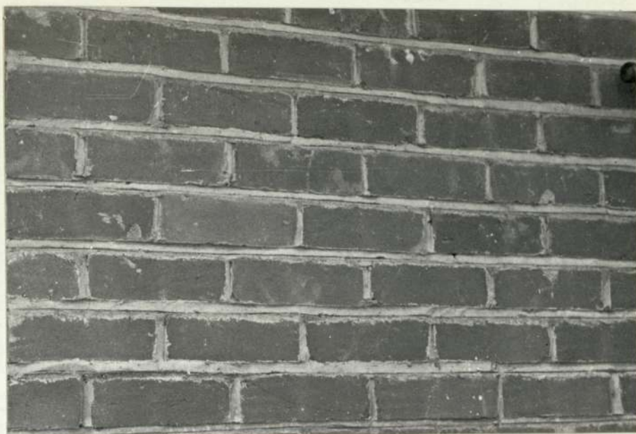
Plate 18.6 Example of poor workmanship in wall
