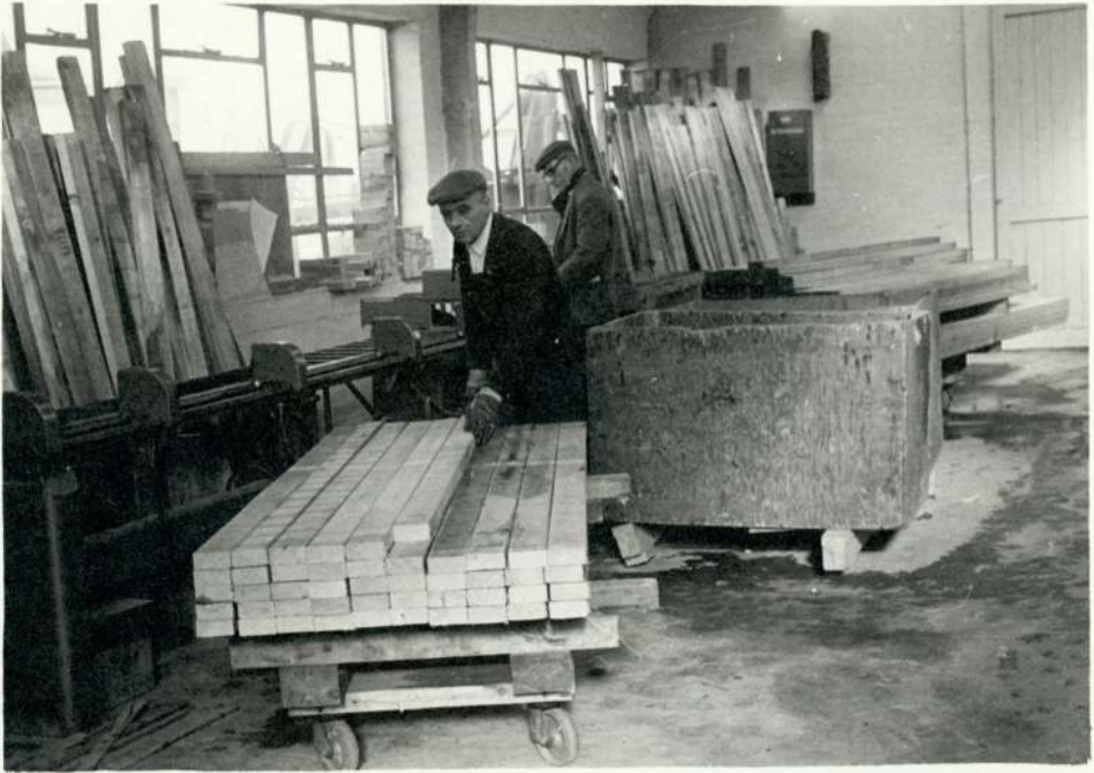
Fig. 6.5 Panel studs being cut on an automatic cross cut
