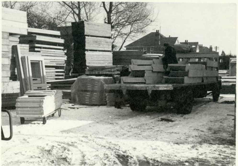
Fig. 6.10 Joinery sets being loaded to flat base lorry
