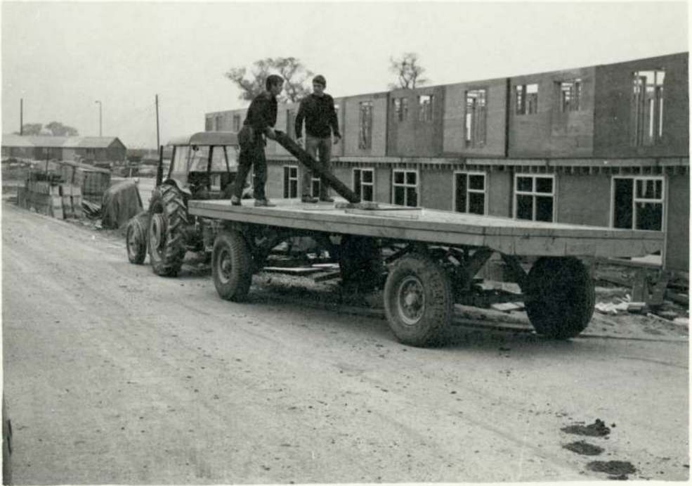
Fig. 6.23 Tractor and trailer used for site transportation
