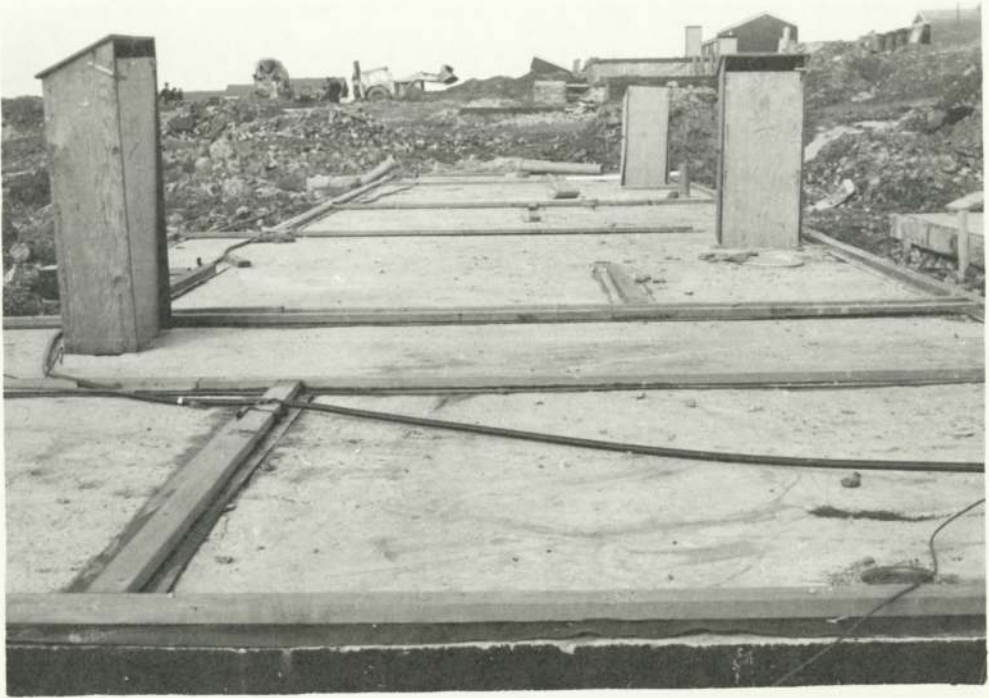
Site slab with box terminals for electrical connections
