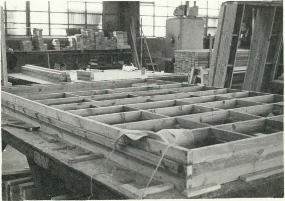
Bottom panel being used as template for a set of panels
