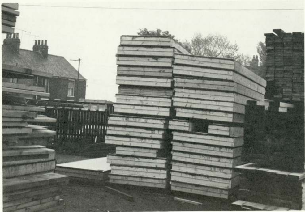
Storage of floor units prior to transportation (in block lots)
