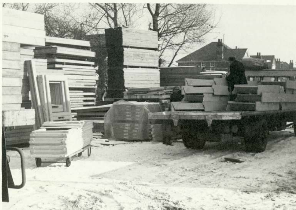
Fig. 6.4 Panels and timber in open storage
