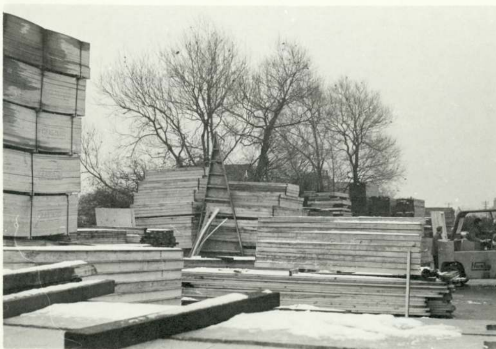
Fig. 6.3 Storage of plywood and large panels
