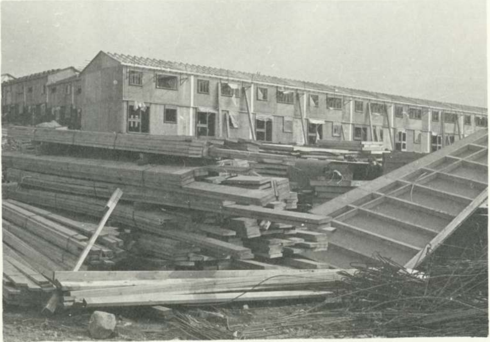
Floor joists bundled in house lots
