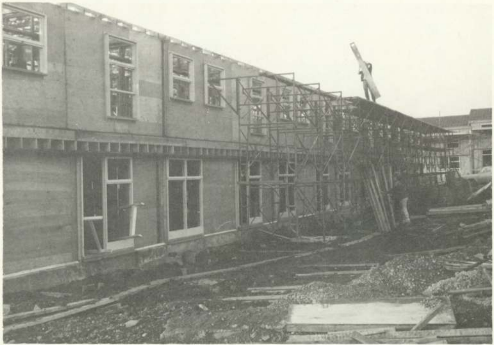
Fig. 7.38 Independent scaffolding with extension brackets (Kwik-stage type)
