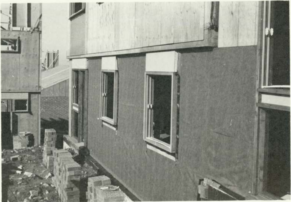
Timber frame complete showing overhang of upper storey
