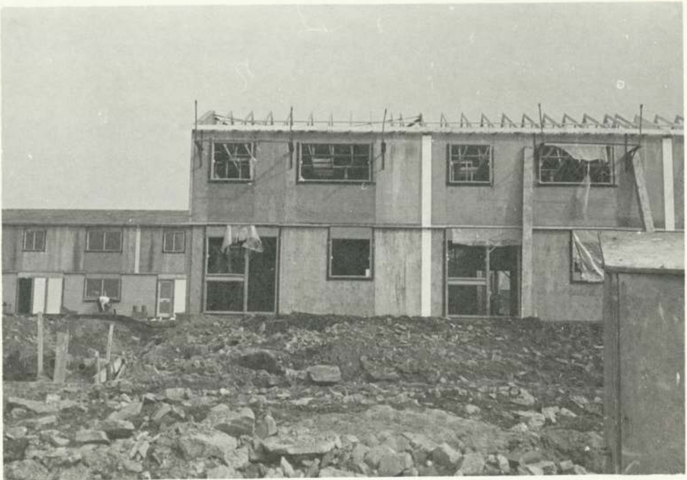
Roof trusses fixed and supported by wind bracing
