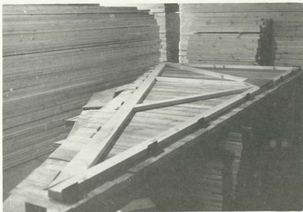
Completed roof truss on bench jig Fig. 6.32
