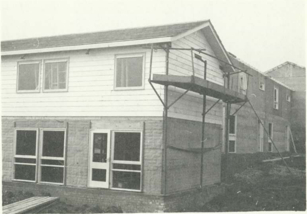
Specialist scaffolding bolted to gable end for cladding operations.
