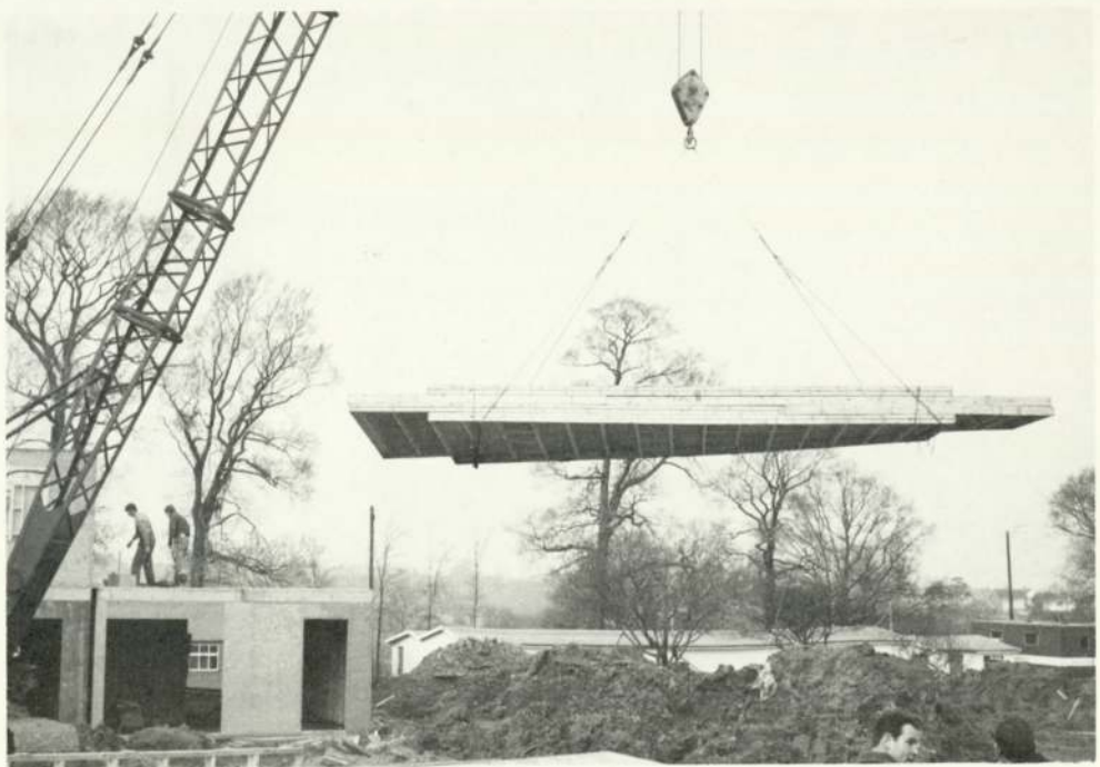
Fig. 7.14 Panels twisting under stress of lifting
