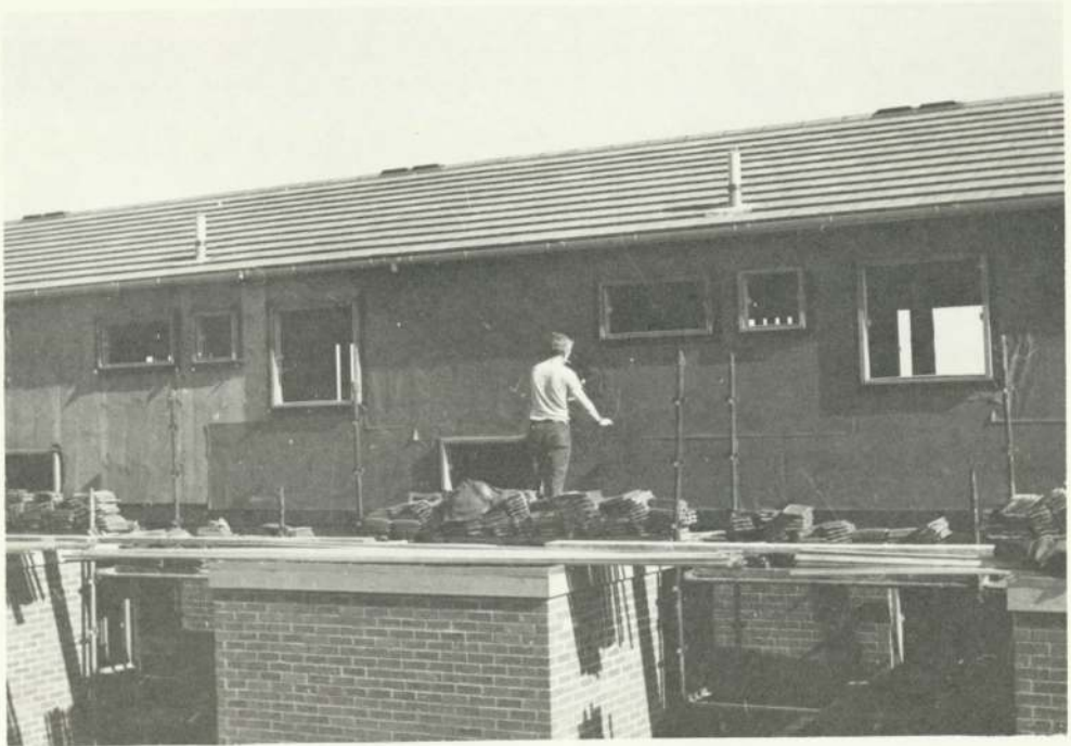
Moisture barrier being fixed prior to vertical tiling
