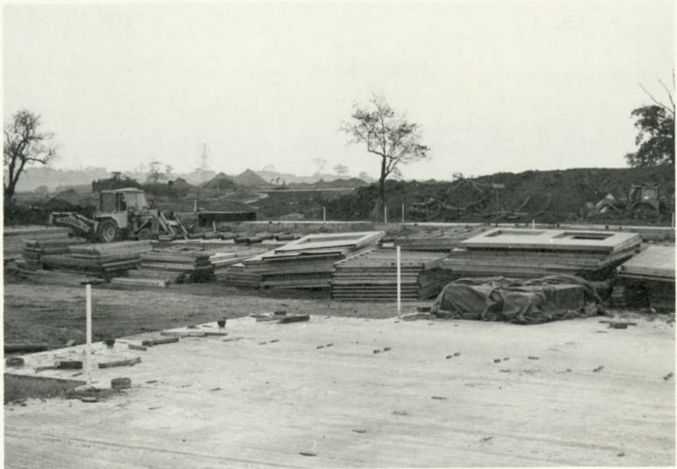
Fig. 6.24 Panels stacked alongside slab for erection
