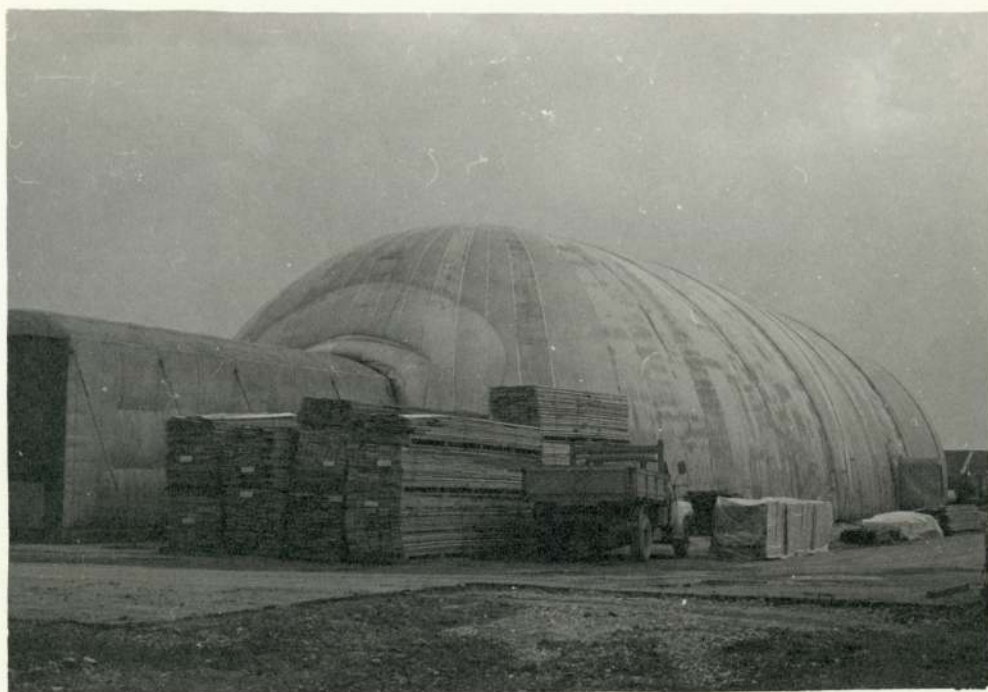
Fig. 6.42 General view of Air House showing passage entrance for fork lift trucks
