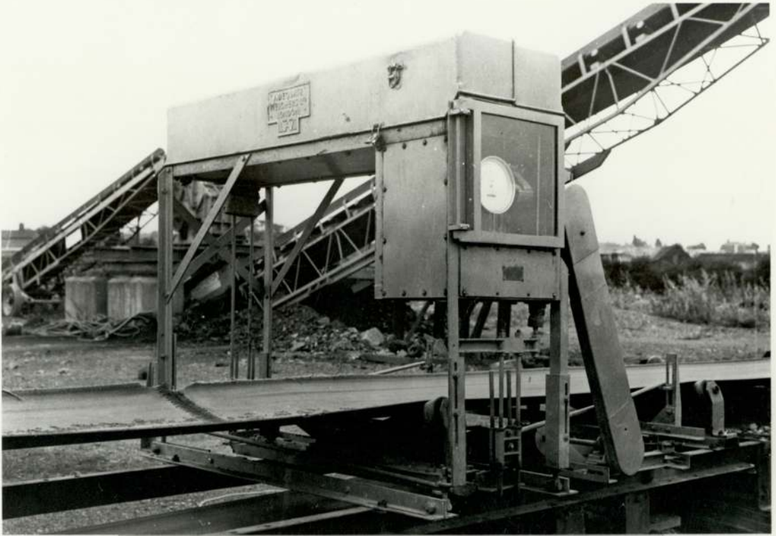
FIG 14 AUTOMATIC WEIGHING MACHINE BETWEEN BUNKER & STOWER
