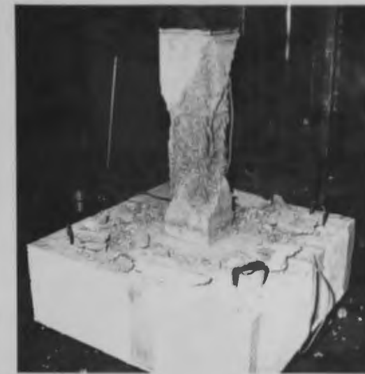
View of specimen after breaking off the loose concrete
