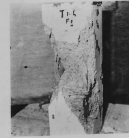
View of column after removing the loose concrete
