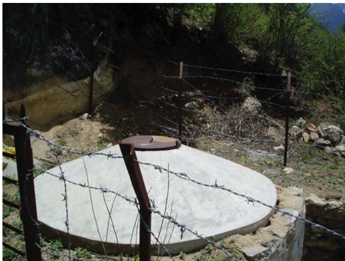
Picture 9: Reservoir tank for drinking water system, Dundafaya
