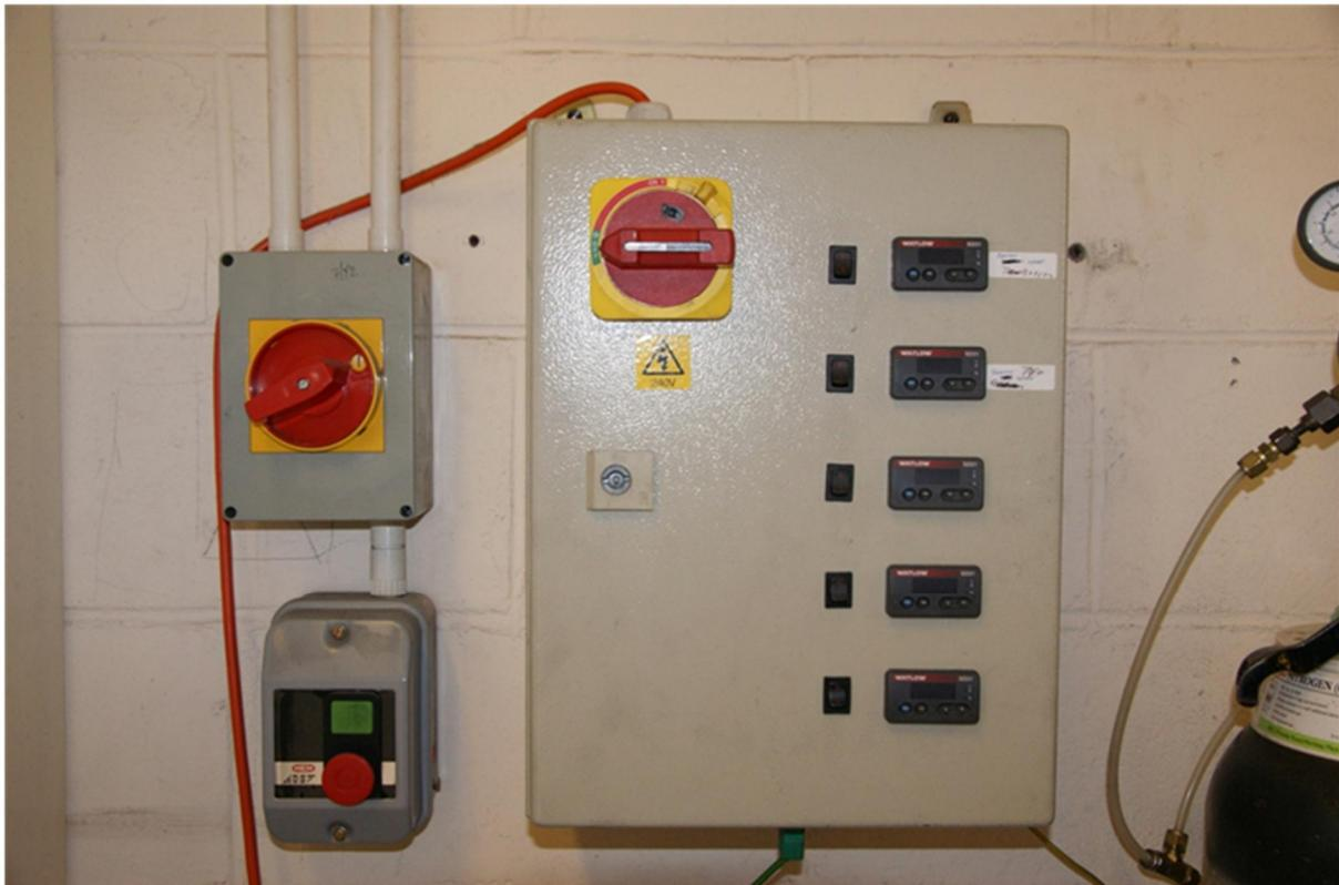
Figure 6-8 Watlow multizone temperature controller
