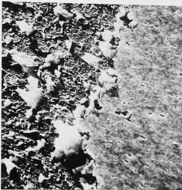
Fig.9. Edge of "corrosion circle". Corrosion products present where electroless nickel had been attacked and torn ABS surface where the coating had still been bonded to the substrate. Plastics grade X, process sequence B, coating system No.4., 16 hr CASS test. Magnification x 1300.
