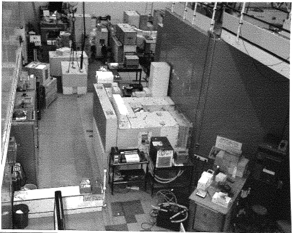
Plate 26 – Concrete Shielding to Cavity
