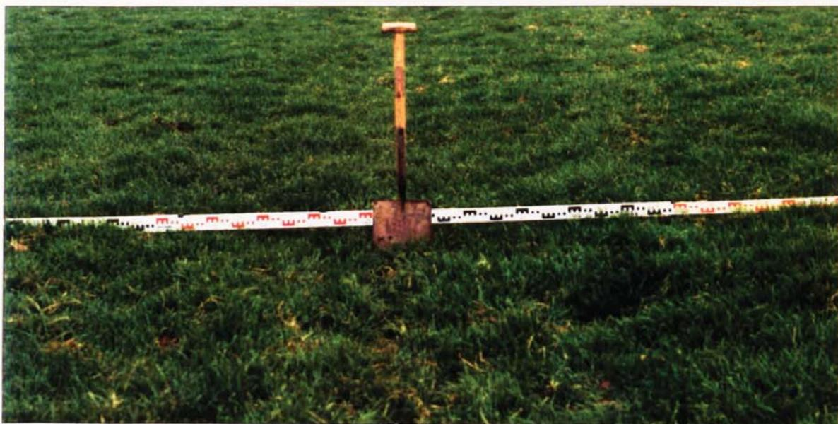
PLATE 7.14 Depression Across the Pipeline between MP19+50 and MP20.
