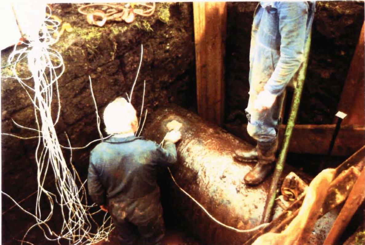
PLATE 7.4 Installation of Thermocouple-Psychrometers at Site A.
