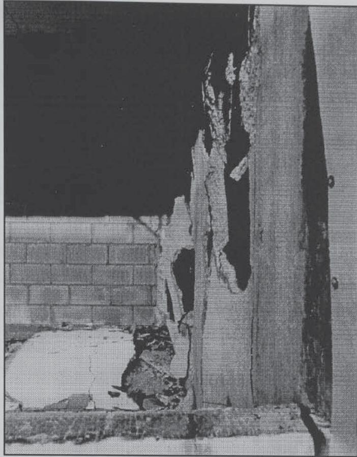
Plate 1.5 Explosive spalling of concrete slabs under real fire conditions
