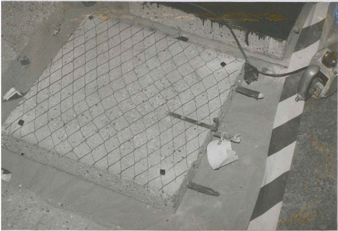
Plate 6.1 Mesh anode fixed to a concrete slab before the application of cementitious overlay.
