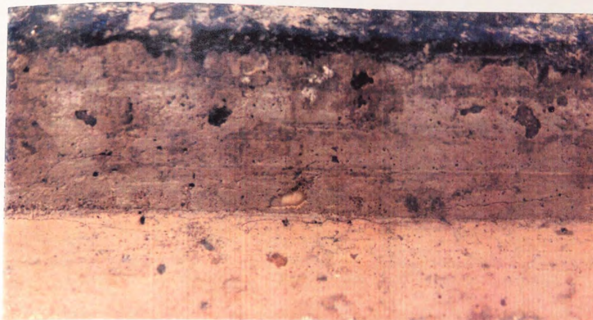
Plate 4.3 - Cracking of Ponding Surface (Sodium Formate) x 1.5 Mag.
