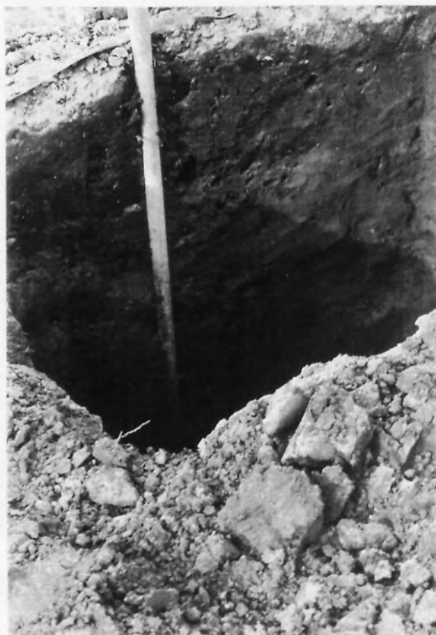
TRIAL PIT AT HEATH HOUSE ACCESS TUBE 4 - 15th April 1980.
