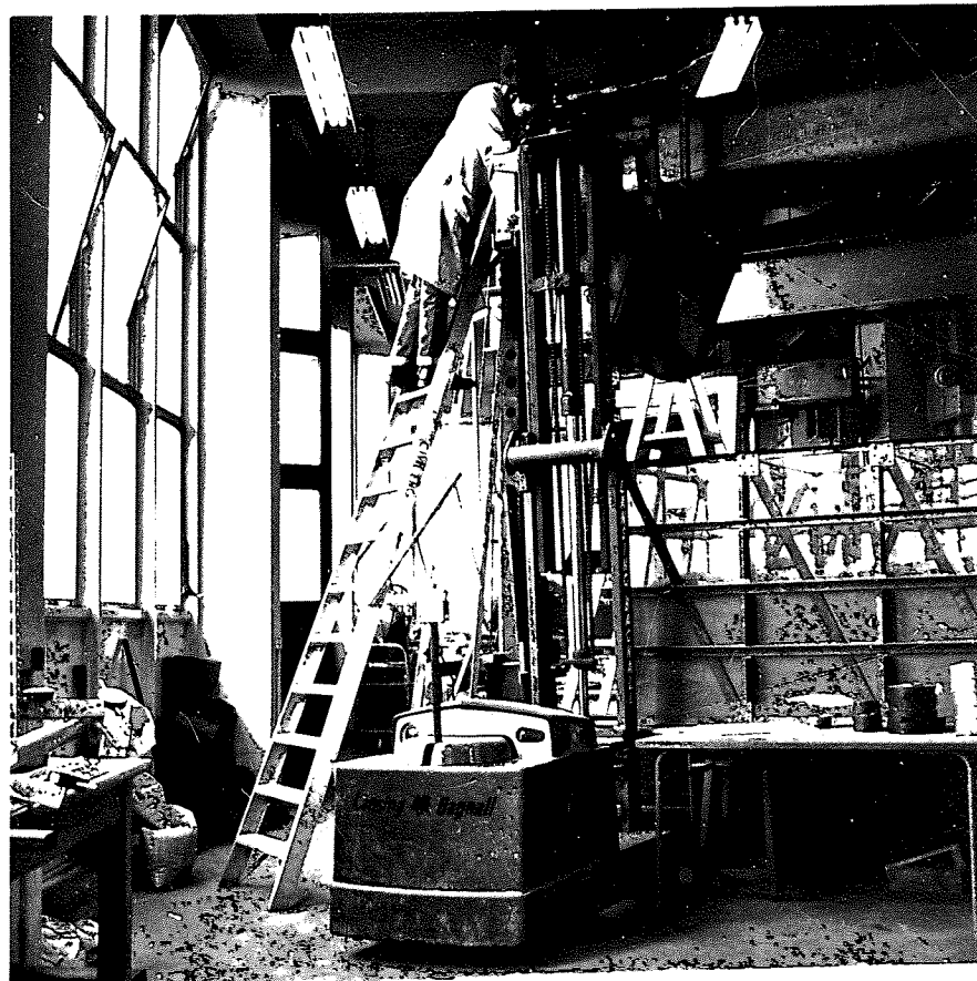
PLATE (5.8b) THE HOPPER BEING ATTACHED TO THE TROLLEY
