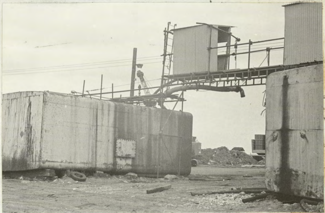
FIGURE 3.8. Temporary Oil and Water Separation Plant. Constructed in a makeshift manner on a landfill site and not complying with the necessary constructional and operational standards.
