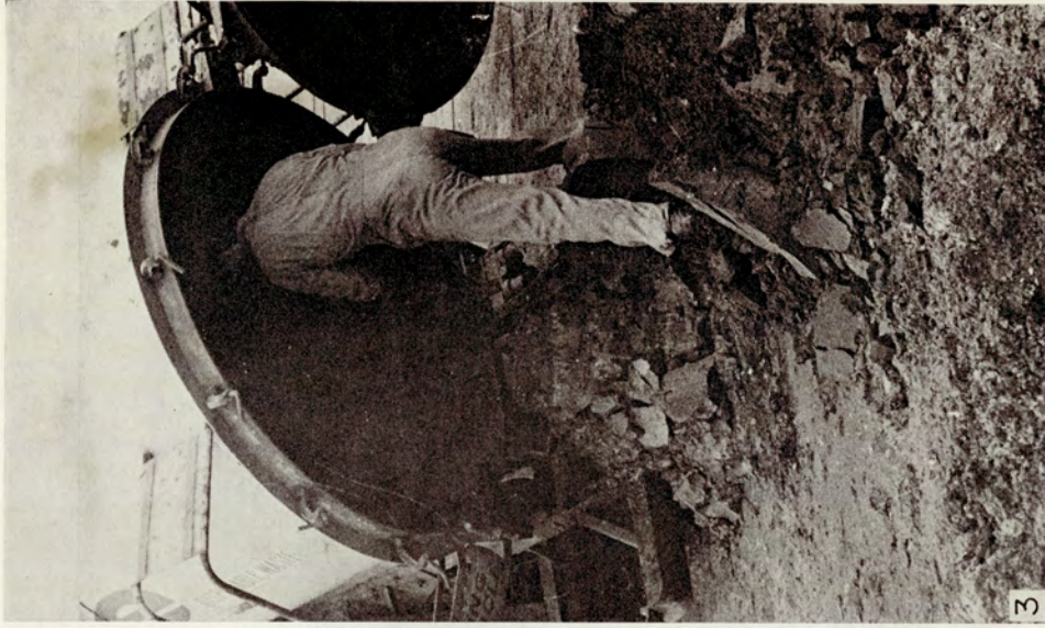
FIG. 2. Operator controlling the discharge of waste into reception pit which is deep enough to present a drowning risk and besides containing a toxic and/or corrosive mixture might give off hazardous gases.
