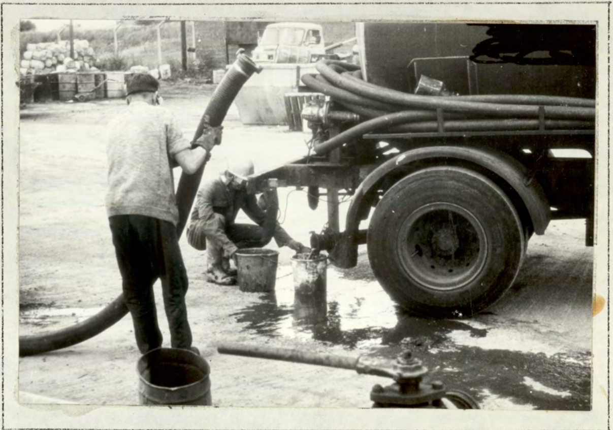
FIGURE 4.2 Discharge pipe connections This shows the drainings from a road tanker being collected subsequent to the dis-connection of the discharge pipeline.
