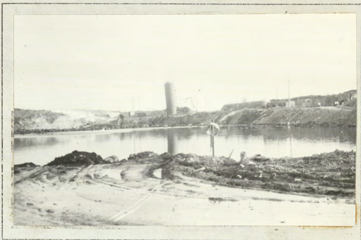
FIGURE 3.9 Landfill into a deep lagoon Also visible is a vertical storage silo which is leaning out of vertical alignment, probably due to settlement of the tipped materials.
