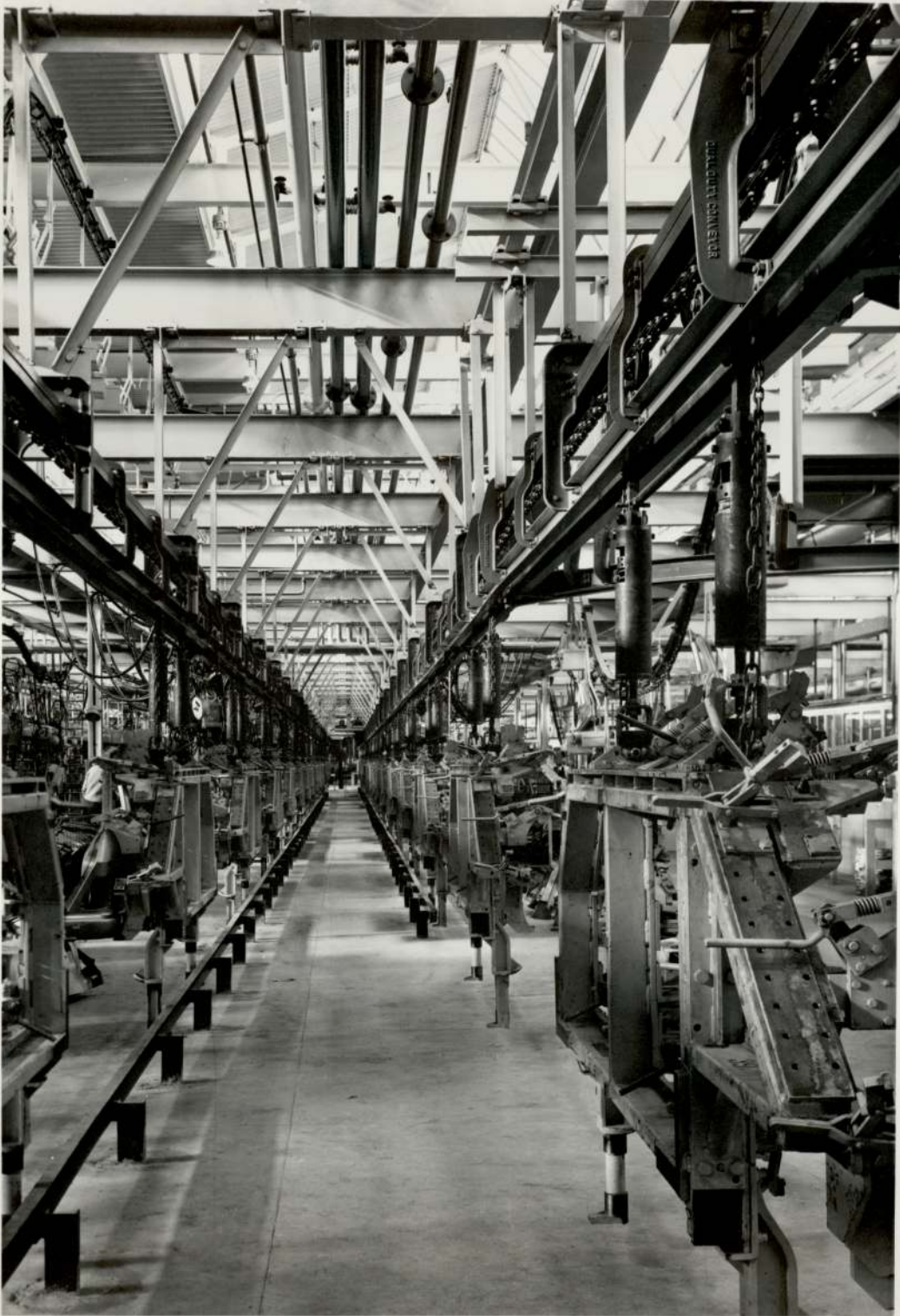
PLATE I SIDEPANEL BUILD - MAXI GATELINE
