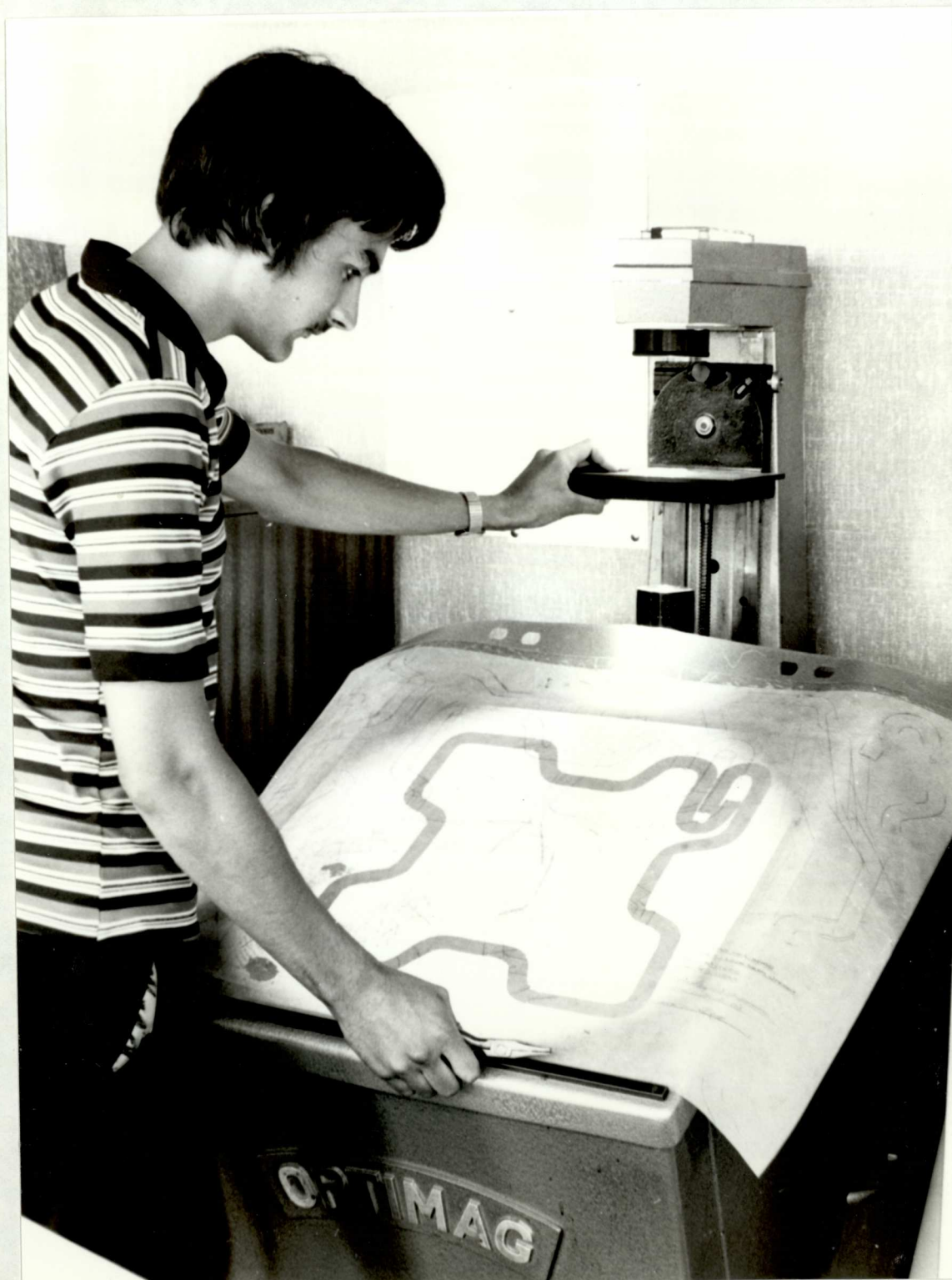
Plate 2.4 PRODUCTION OF THE WIRE-TEMPLATES ON A SHADOWGRAPH PROJECTOR
