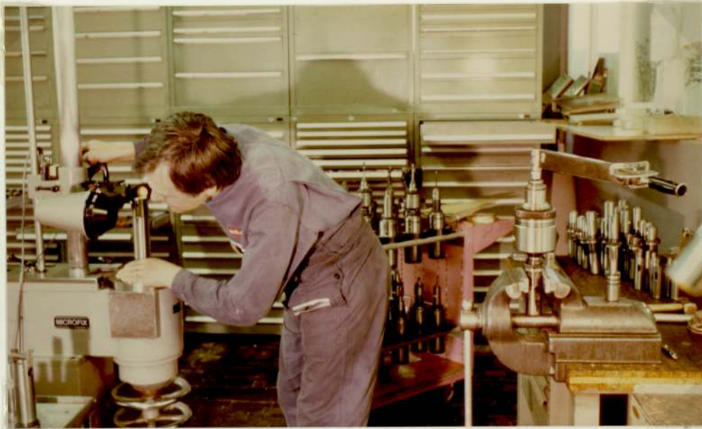
174b BORING-BAR PRESETTING
