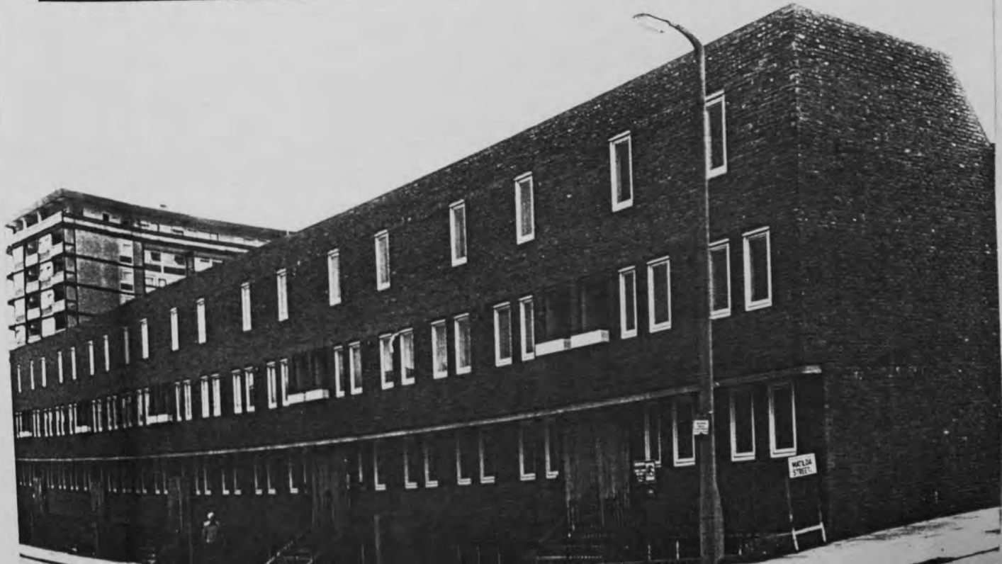
THE G.L.C.'S NEW INFILL DEVELOPMENT ON THE NORTH SIDE OF COPENHAGEN ST. BETWEEN MATILDA ST. AND COPENHAGEN ST. fig. 4.39
