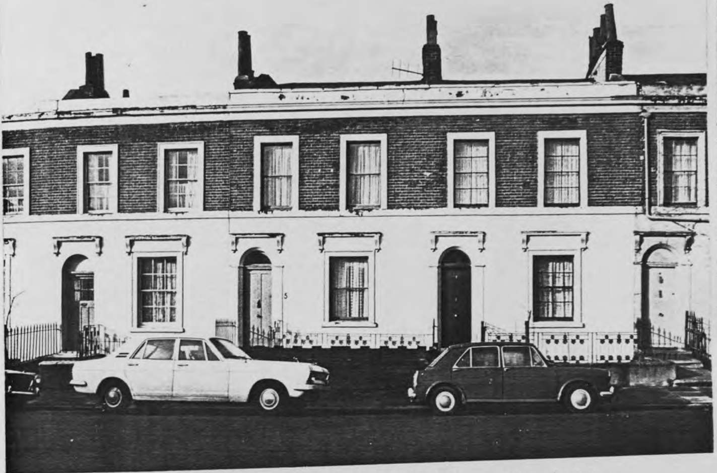
A VIEW OF THE SOUTH END OF HEMINGFORD ROAD fig. 4.10 LOOKING SOUTH, THE WEST TERRACE (TO THE RIGHT OF THE PHOTOGRAPH) HAS SINCE BEEN DEMOLISHED
