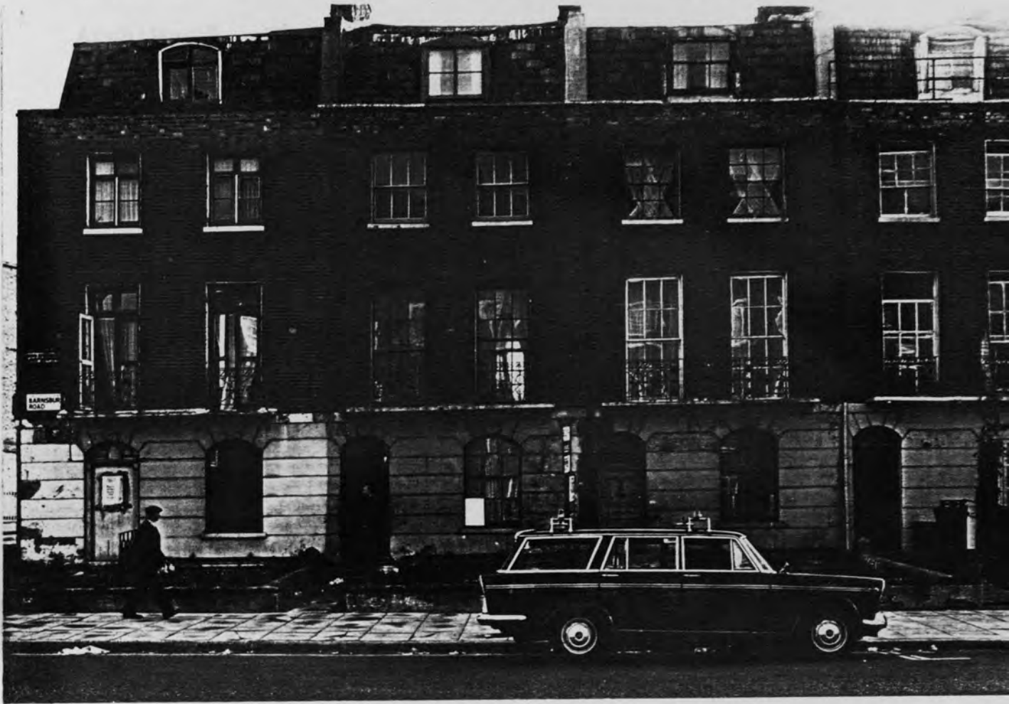
56-62 BARNSBURY ROAD BEFORE CONVERSION WORKS fig. 5.37 WERE COMMENCED IN JANUARY 1972
