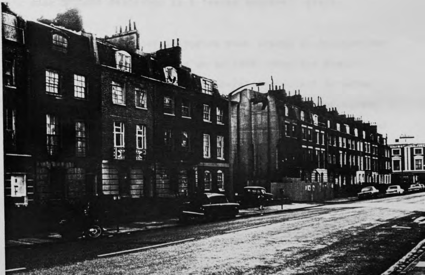
18-48 BARNSBURY ROAD BEFORE CONVERSION WORKS fig. 5.38 WERE COMMENCED IN JANUARY 1972
