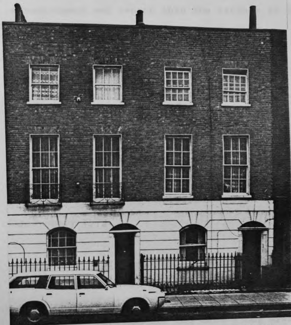
PHOTOGRAPH SHOWING BALCONIES & RAILINGS TO HOUSES 1-23 COPENHAGEN STREET IN 1976
