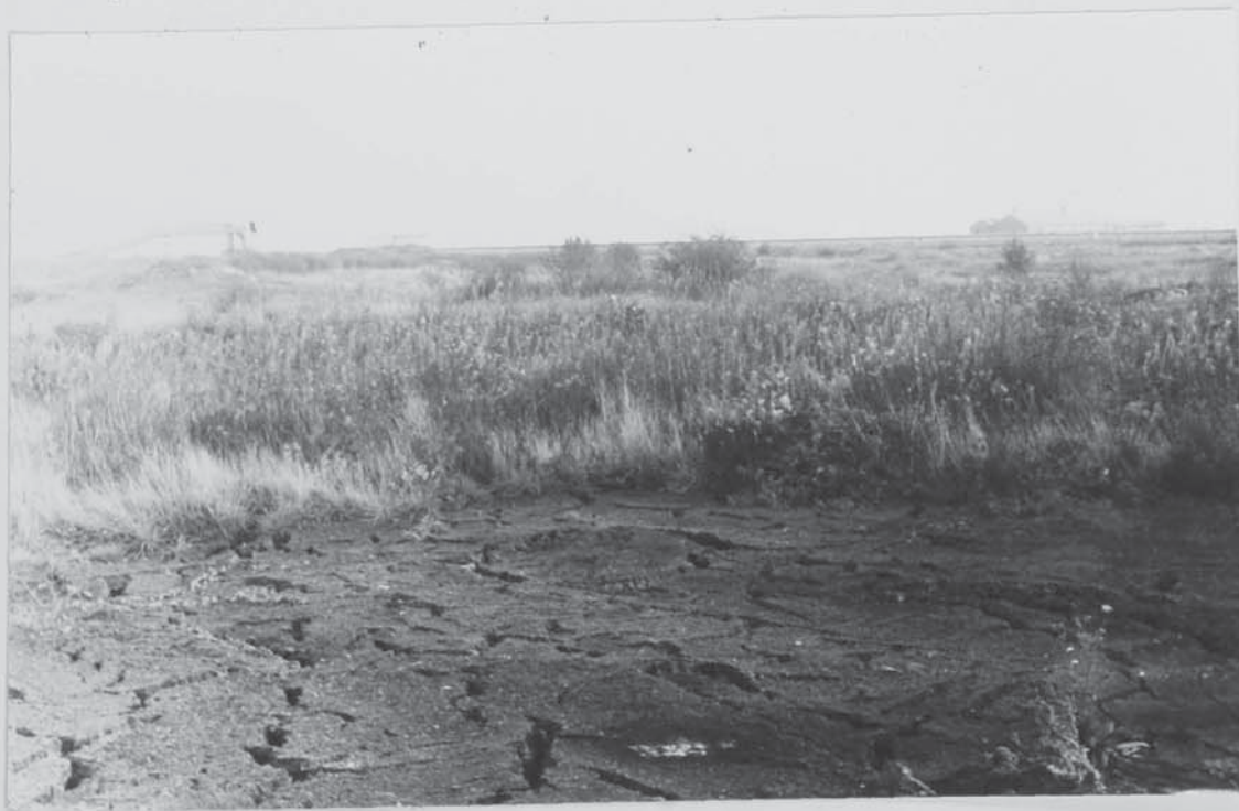
Plate 4.2. PMB six months after deposition showing fissures developing as the material contracts.
