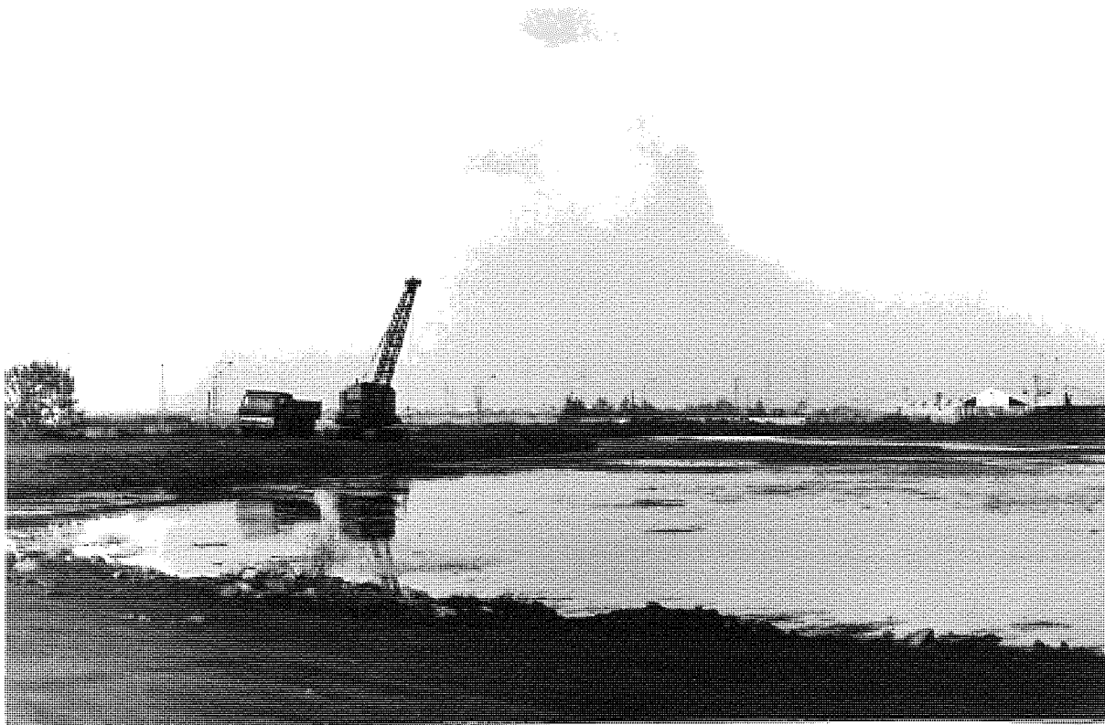
PLATE 1.1 THE PRIMARY TREATMENT OR SETTLING LAGOON.
