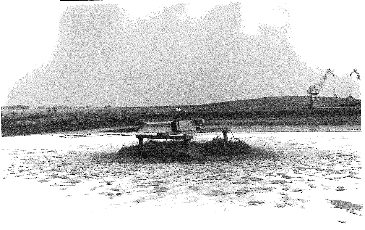
PLATE 1.4 SECONDARY TREATMENT OF THE MILL EFFLUENT IN ONE OF THE AERATED LAGOONS.
