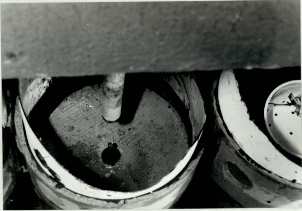
Plate 13. Pilot filter system surface covering modification
