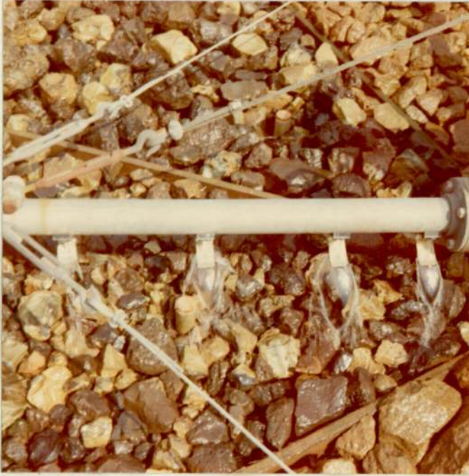
Plate 4.9 Distributor Jets and Splash Plates.
