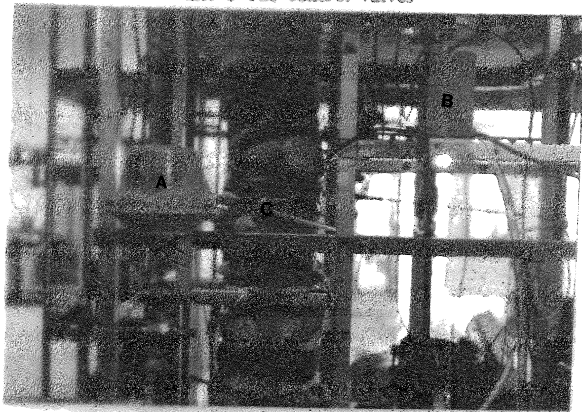
Plate 2 The control valves
