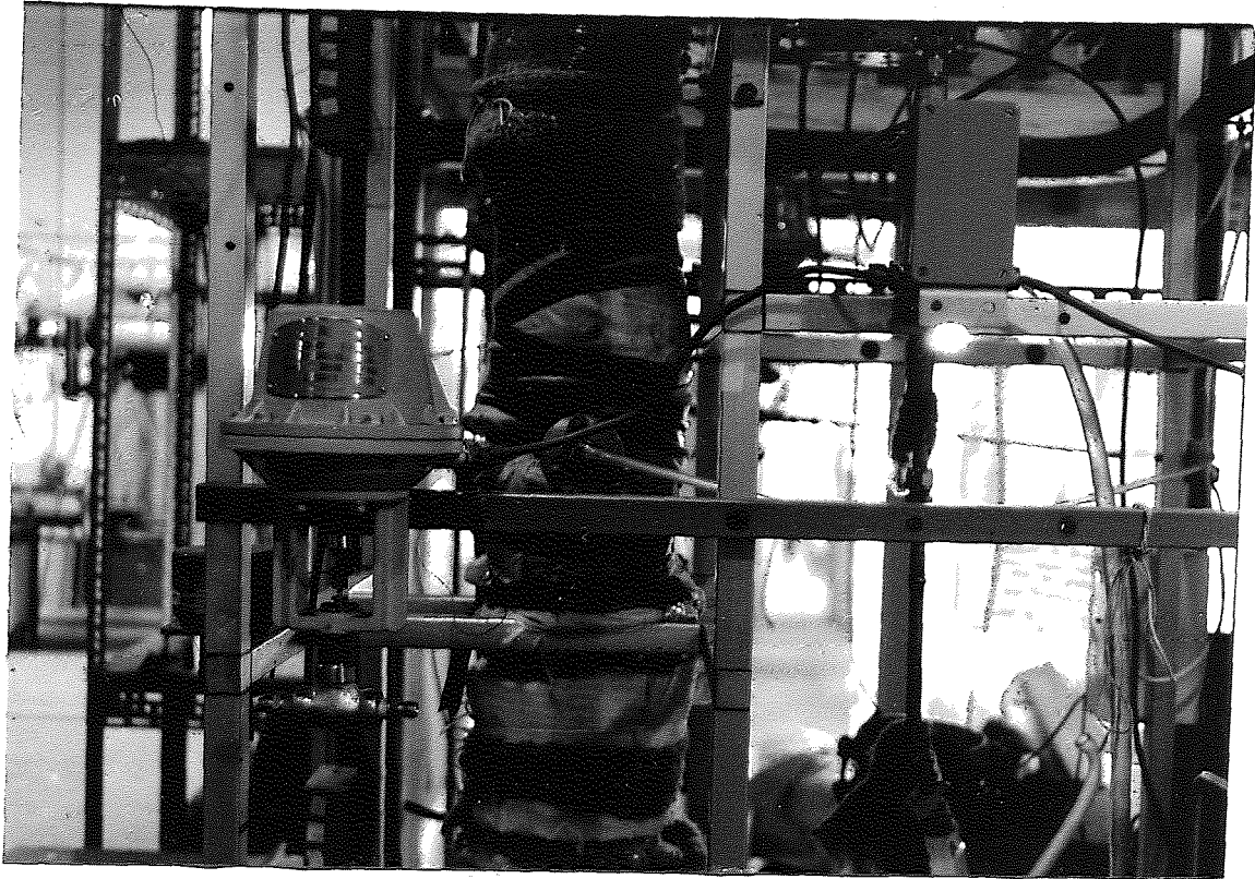
Plate 2 The control valves
