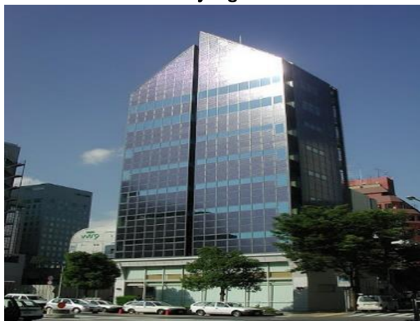
BIPV Solar Facade
