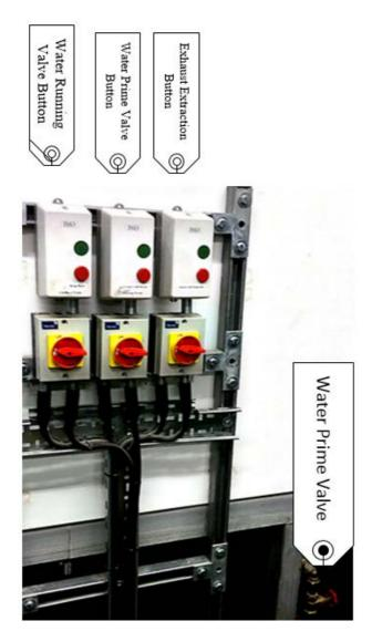
Figure 46: Water and exhaust extractions control keys.
