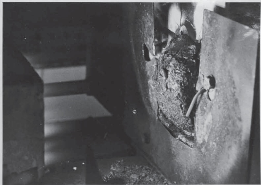
Plate 6.2 : Typical restricted char, around 20 mm; obtained after around ten minutes in a test at 750° - 800°C.
